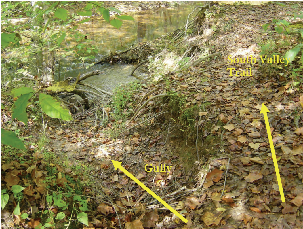
Figure 7. Gullying along the South Valley Trail. Photograph by Trista L. Thornberry-Ehrlich (Colorado State University).
