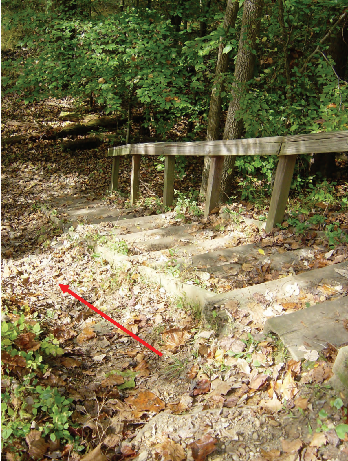
Figure 3. Erosion from foot traffic along the South Valley Trail. This stairway was intended to reduce erosion of the steep slope but its purpose has been undermined by off-trail hiking. Photograph by Trista L. Thornberry-Ehrlich (Colorado State University).
