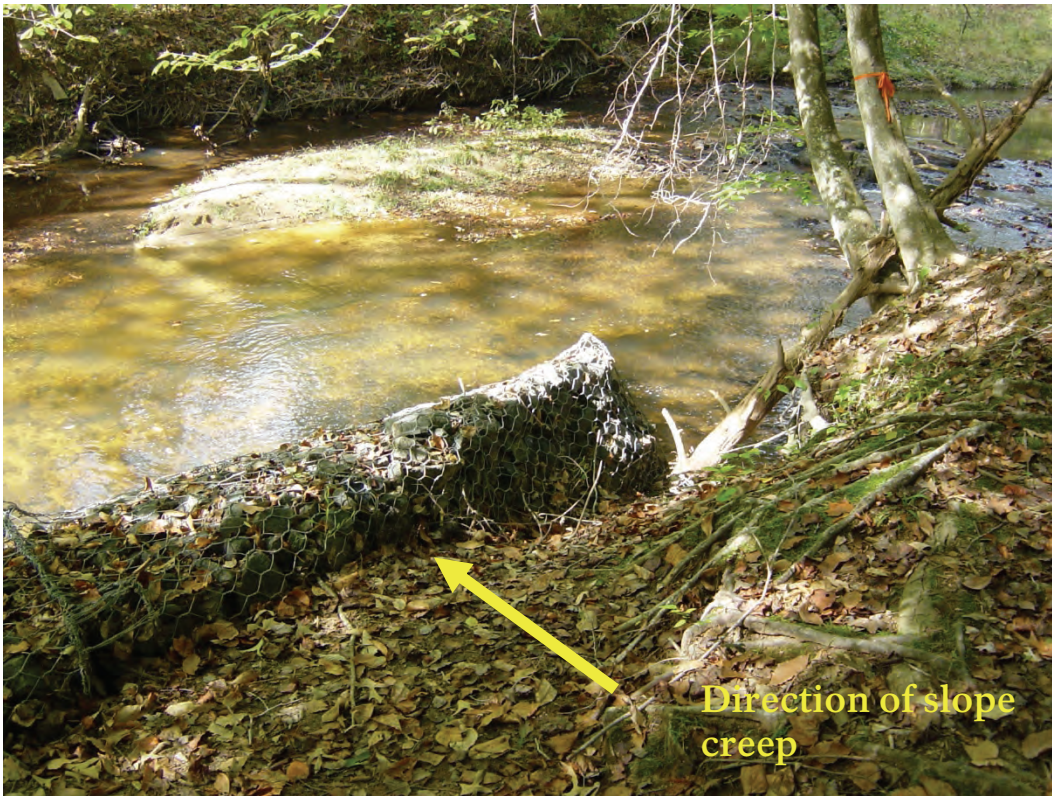
Figure 5. Top-down view of a gabion along the shoreline of South Fork Quantico Creek. This image shows the toe of the slope pushing the gabion into the stream and undermining the trail along the top of the gabion. Photograph by Trista L. Thornberry-Ehrlich (Colorado State University).
