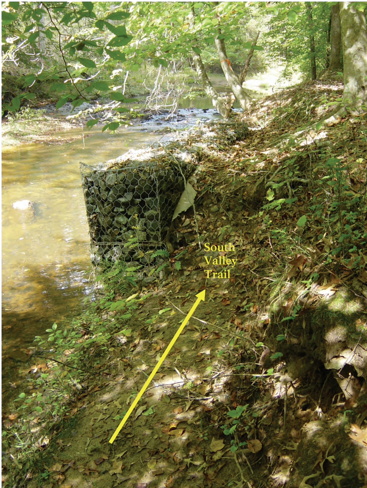
Figure 4. A buttress along South Fork Quantico Creek is intended to prevent erosion of the South Valley Trail (foreground); however, slope creep from the undercut slope above has pushed the buttress out of alignment and is compromising visitor safety along trail. Photograph by Trista L. Thornberry-Ehrlich (Colorado State University).
